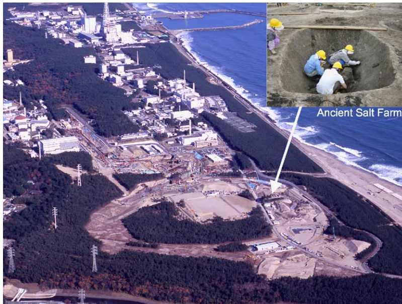
Fig. 3. View from the sky of the construction area.
