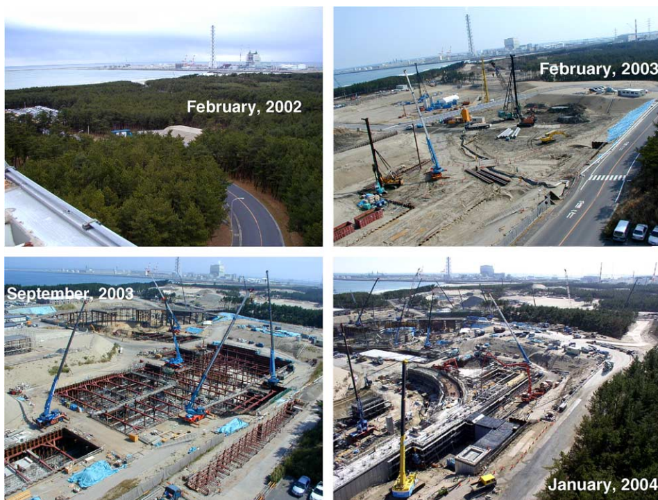
Fig. 5. Progress in the 3 GeV area.
