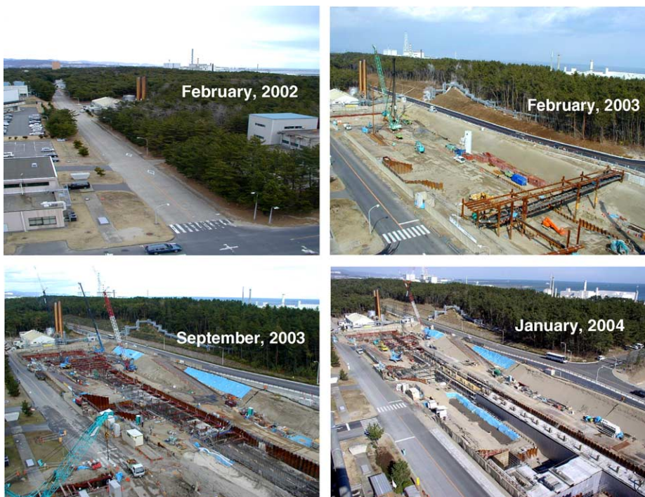
Fig. 4. Progress in the Linac area.
